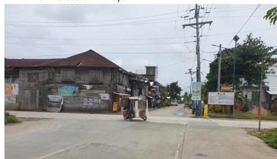
KM 117.3 Intersection in Dapa
